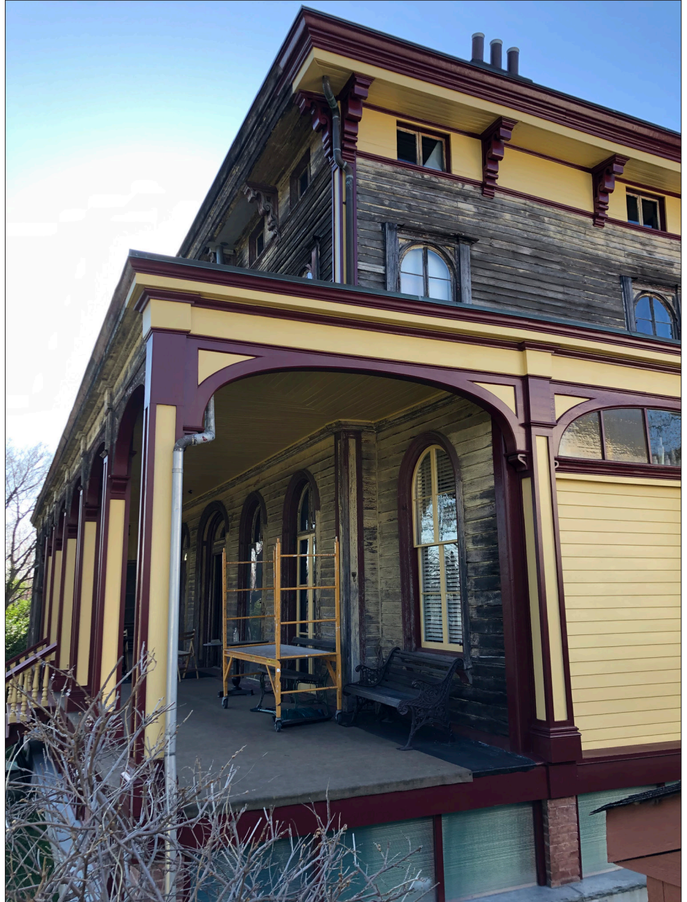
An example of the restoration in progress.
