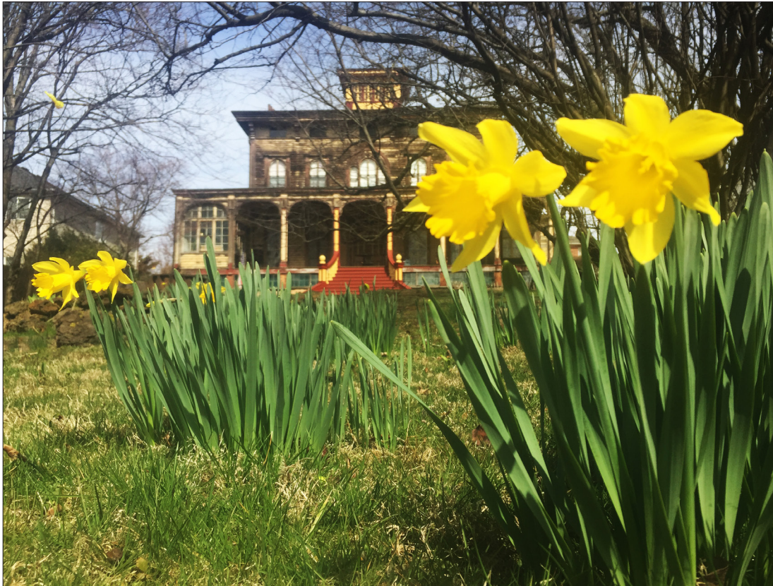
A view of the front of the Gustav Mayer House, from Richmond Road.
